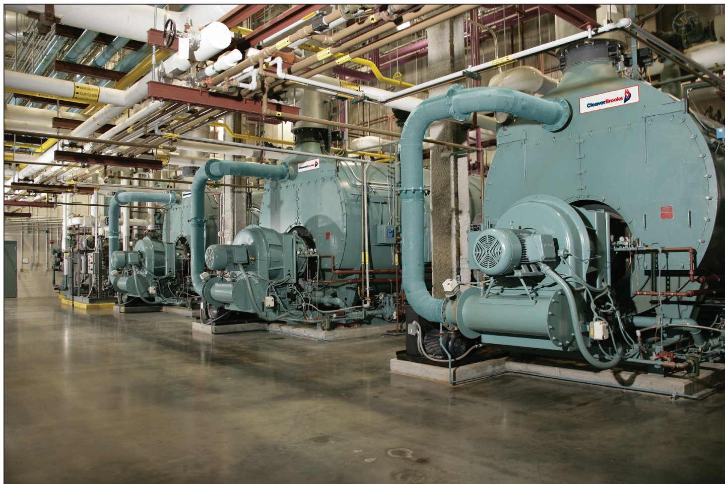
Charlotte Medical Center installation of three ICB firetube boilers
