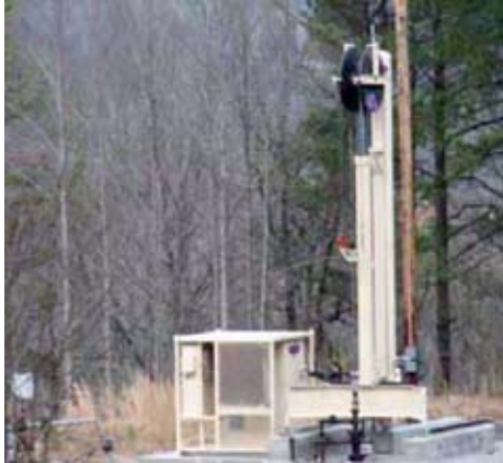
DynaPump Model 7 operating in Alabama
