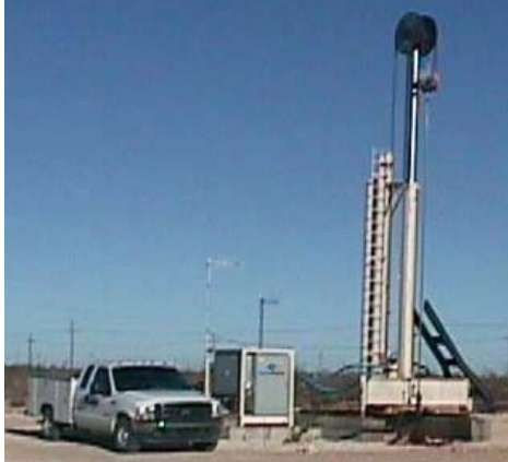
DynaPump Model 9 operating in West Texas
